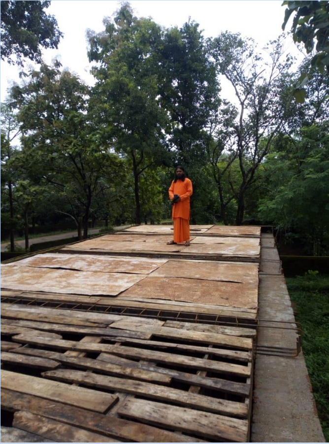
Steel rod binding and Shuttering work for Roof concreting of Atulananda Bhavan
